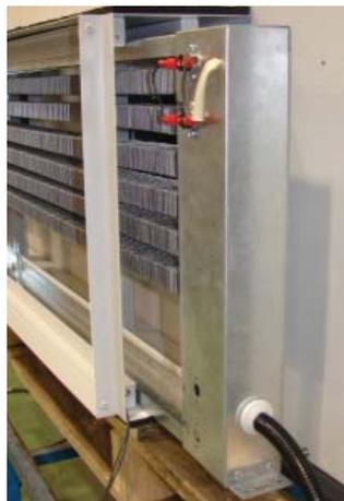
Step 3: insert the hose through the hole made for the connection in the electric panel.
